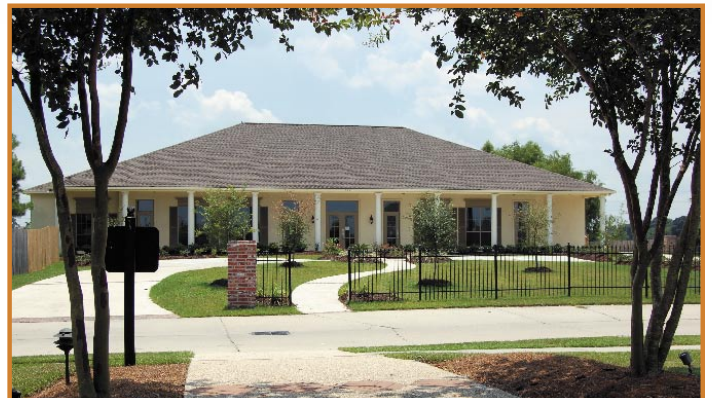
The Greens' New Clubhouse...putting on the finishing touches!
